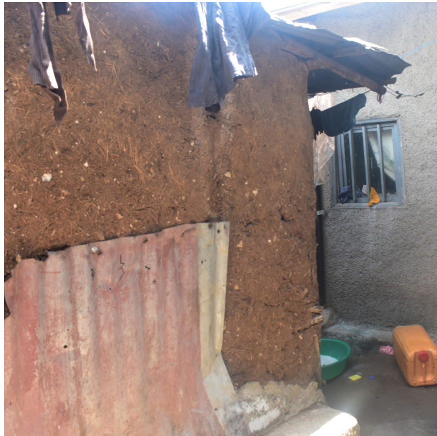
A traditional way of wall construction used throughout Ethiopia is Chika: a load-bearing wall with eucalyptus wood as frame structure and mud as infill. Some people opt to also add a layer of cement plaster on the mud surface as a water barrier.
