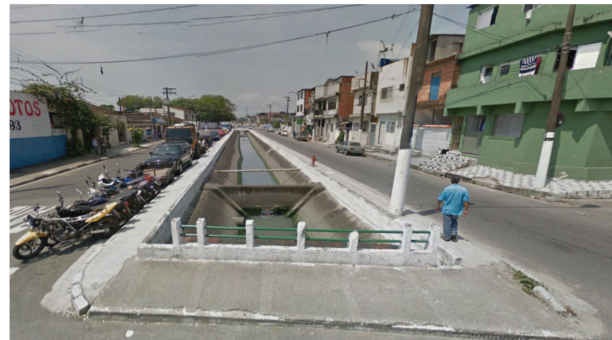
A canal in the Zona Noroeste of Santos, with a lack of green. source: Google Streetview
