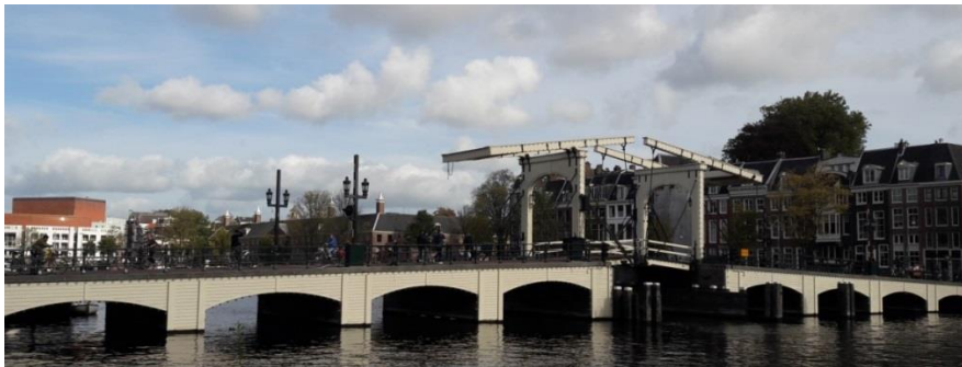
Figure 16 Magere Brug, an Amsterdam landmark
