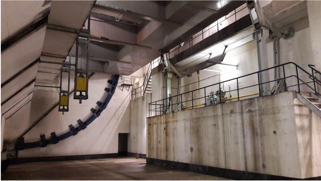
Figure 11 Bridge 485 – Oosterdoksbrug basement, revealing the counterweight and safety works
