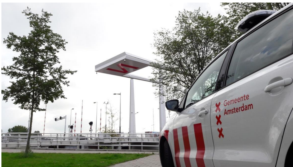
Figure 2 Amsterdam, bridge 491 - Bascule bridge
