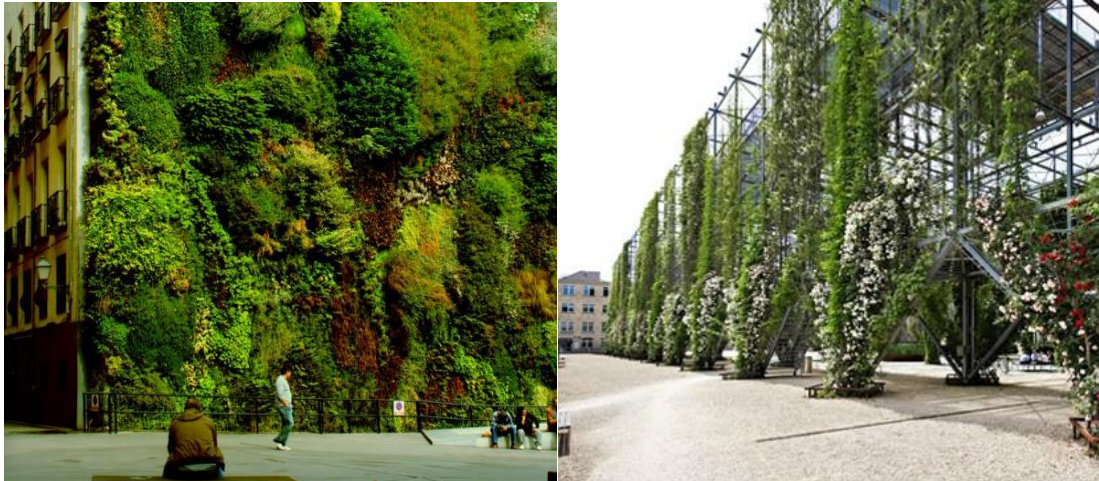
Figure 62 Left: vertical garden, CaixaForum Madrid (source: blogspot.com) and right: green façade (source: MMA architecture)
