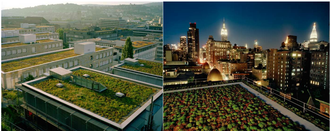
Figure 58 Left: Green roofs in Stuttgart and right: New York City (source: nationalgeographic.com)
