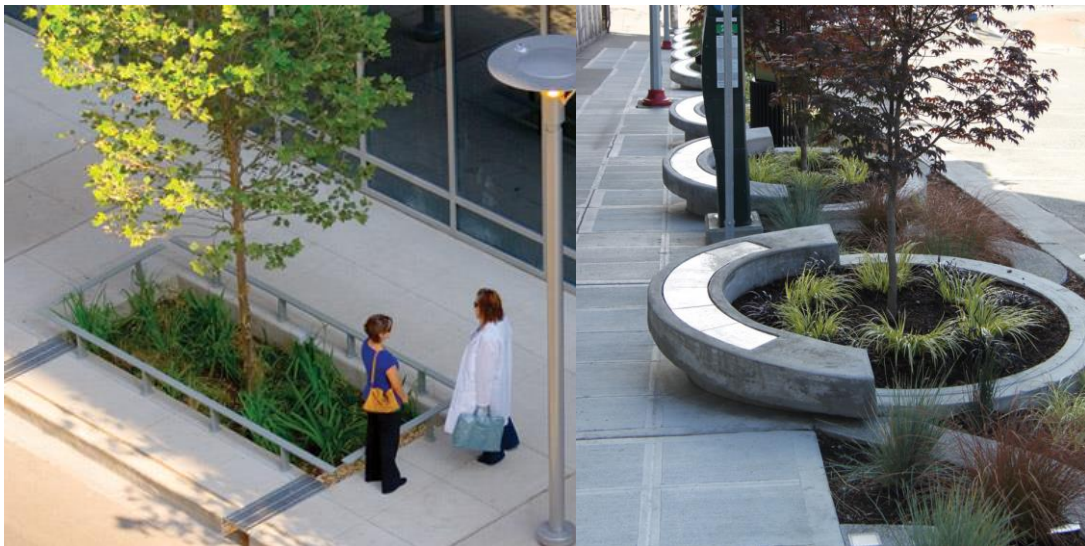
Figure 55 Storm water Infiltration/flow through Planters in Illinois (left) and Seattle (source: spur.org)
