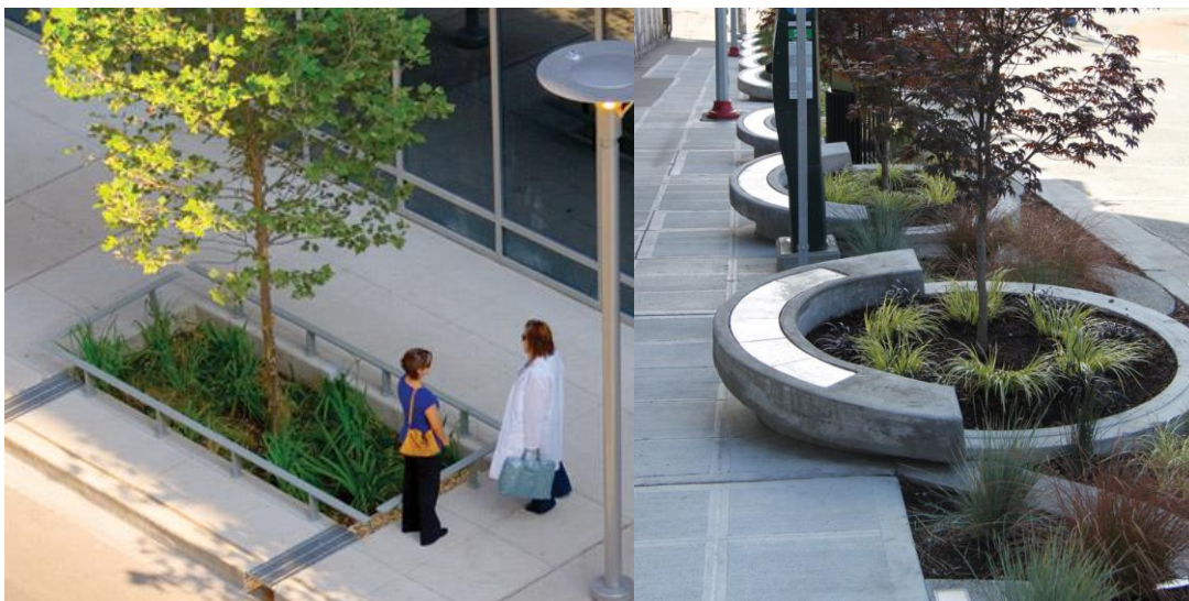
Figure 55 Storm water Infiltration/flow through Planters in Illinois (left) and Seattle (source: spur.org)
