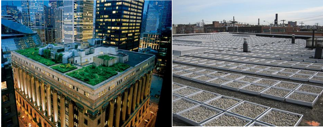
Figure 57 Left: Green roof, Vancouver (Source: nationalgeographic.com) and blue roof (water roof) (source: reducerunoff.org)
