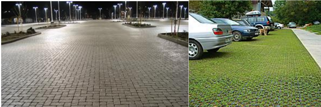
Figure 56 Permeable Pavement Vancouver (source: blur.org)
