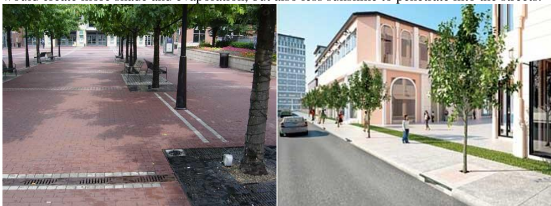
Figure 68 Left: storm water trees Ohio (Source: continuingeducation.construction.com) and right: impression of storm water trees with subsurface chamber (Source: waterworld.com)
