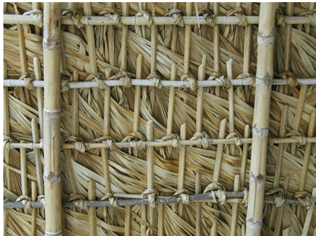
Bamboo and thatch roof connection
