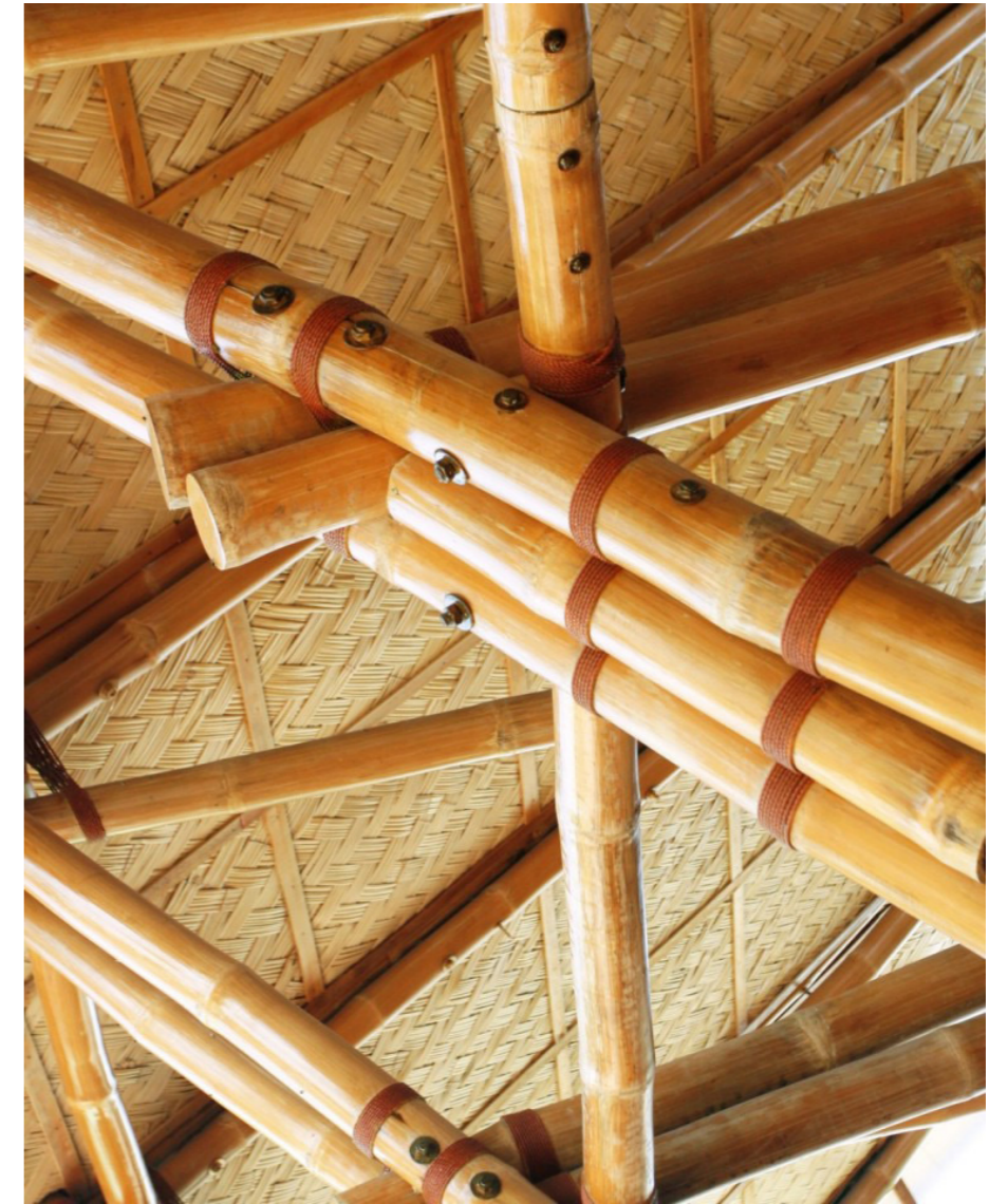
Bolted and Lashing Connection ref: http://constructpix.com/?attachment_id=20
