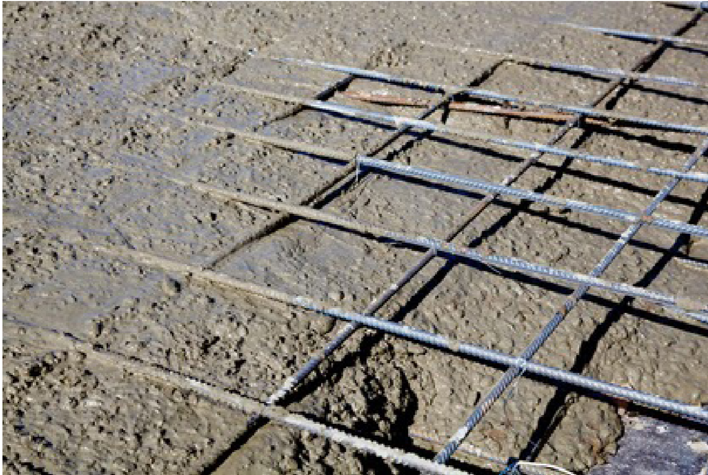
Steel Reinforced Concrete
