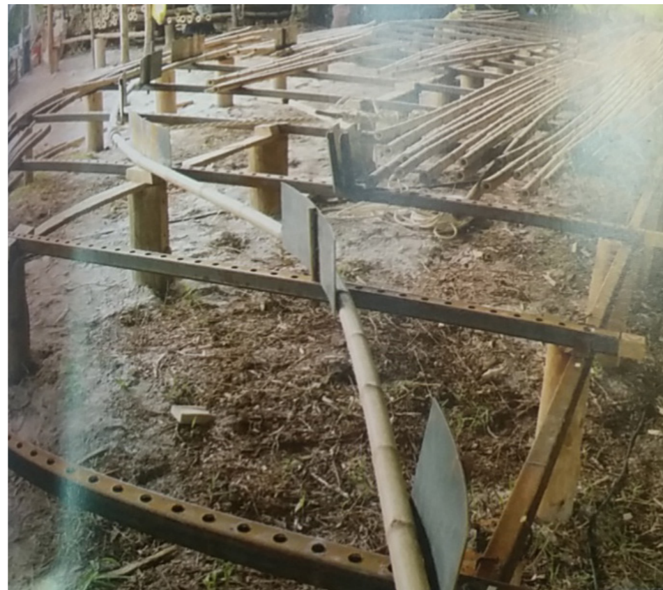
Bamboo bending grid system ref: 24H Architects
