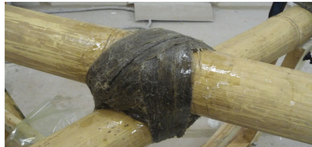
Bamboo connection using composite rope ref: (Jaap Overal)
