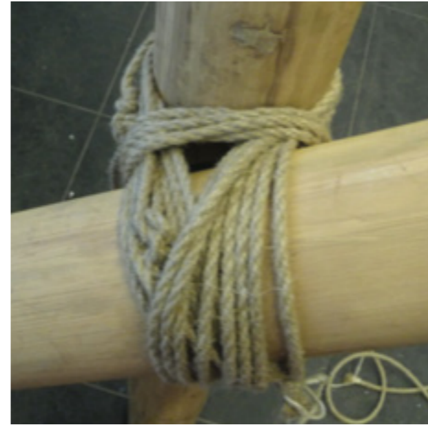
Bamboo connection using hemp rope ref: (Jaap Overal)
