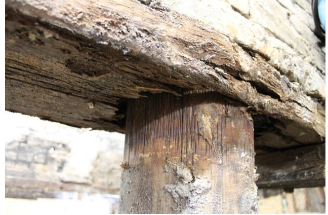
Figure 4.2.2 Rotten pile heads due to decay by fungi ( left ) and rotten head beam punctured by pile head ( top ) (CURNET/SBR, 2007) (Vasiljevski, 2012).
