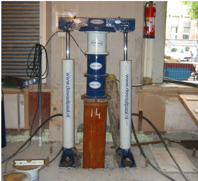
Figure 5.2.4 Jack-down system anchored to the floor (Waalpaal, 2014).
