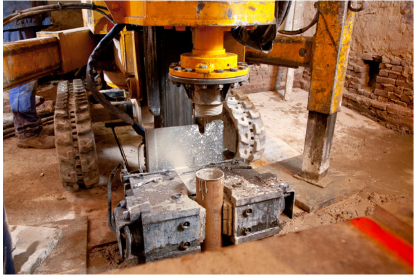
Figure 5.2.3 Screw injection pile (Goorbergh, 2014).
