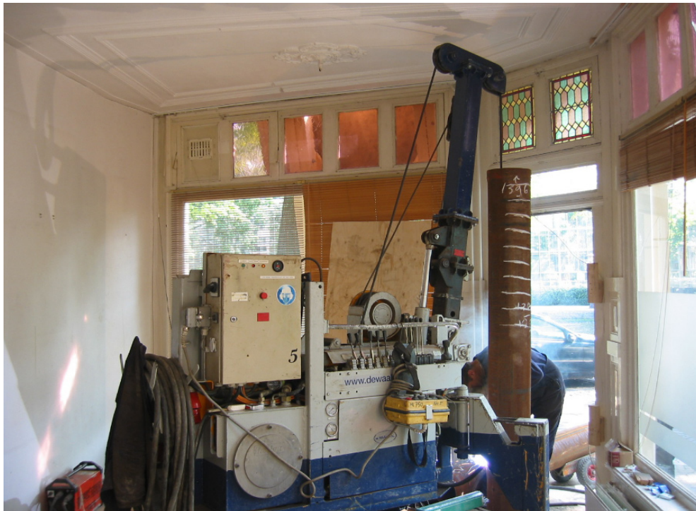
Figure 5.2.2 Bottom driven pile (Waalpaal, 2014).
