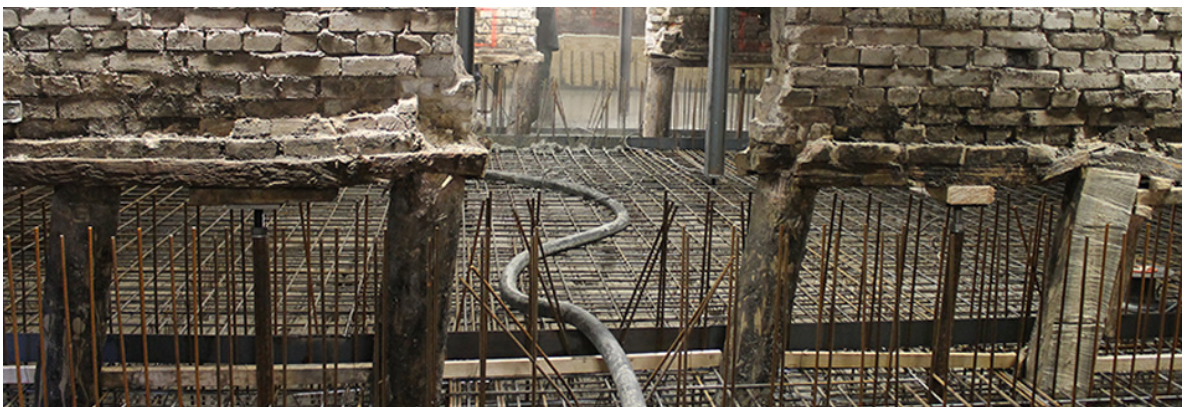
Figure 1.1.1 Construction of new concrete floor slab on piles (Brefu, 2014).
