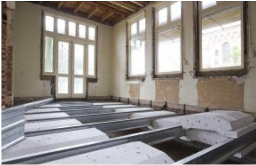
Figure 9.4.1 Beam block composite floor (Bouwwereld, 2014).
