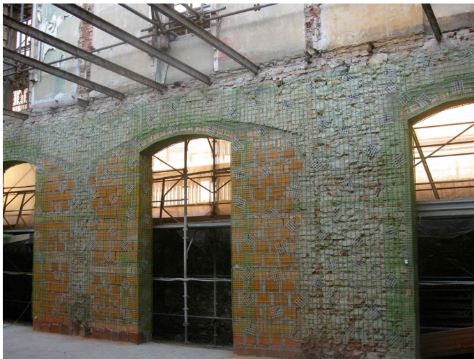
Figure 9.2.2 Example of a FRP mesh that structural reinforces a wall (Fibrenet, 2014).
