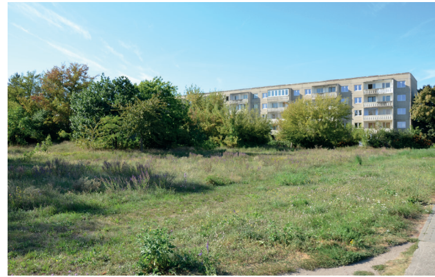
Fig.: 74 Assessment vacant apartment building
