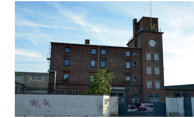
Fig.: 70 Assessment old firehouse
