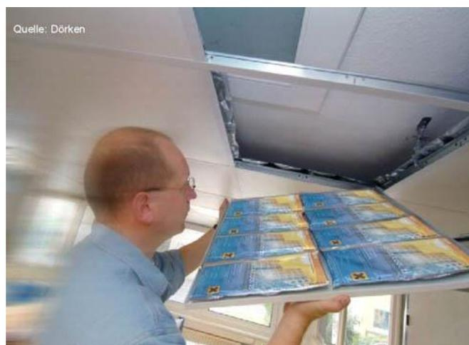
Figure 4.4 PCMs in suspended ceiling configuration
