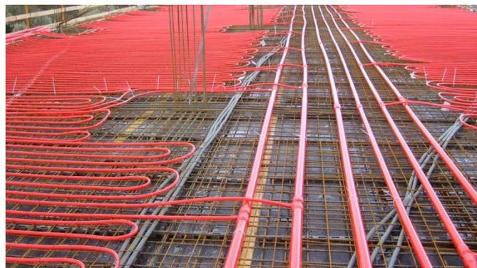
Figure 2.5 Concrete core activation system
