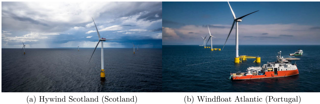
Figure 1.1: The Hywind Scotland (Øyvind Gravås, 2017) and Windfloat Atlantic (Principle Power, 2020) Floating Offshore Wind farms in operation.
