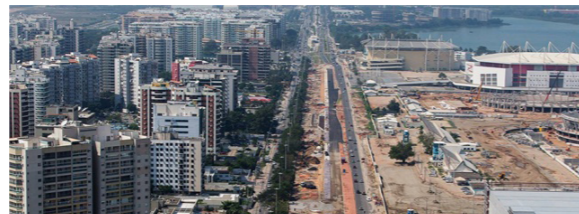
Figure 32 - Construction of the road (retrieved from http://www.metro-magazine.com ).
