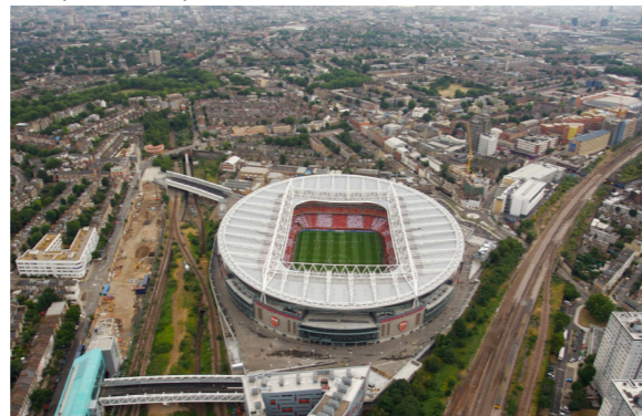
Figure 31 - Emirates stadium aerial picture, left the two crossing bridges to the stadium deck and the major road to the right (retrieved from http://populous.com ).
