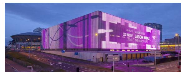
Figure 39 - Ziggo Dome, the screen informs visitors by individually lightning one of the 840.000 led lights (retrieved from http://www.guiding-architects.net ).
