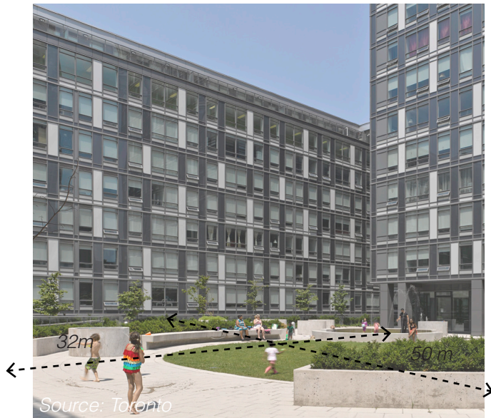
3rd level rooftop courtyard
