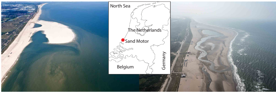
Figure 1.3: Aerial photographs of the Sand Motor after completion of its construction in 2011 (left) and after three years of morphodynamic development (right). Images by Joop van Houdt / Rijkswaterstaat.
