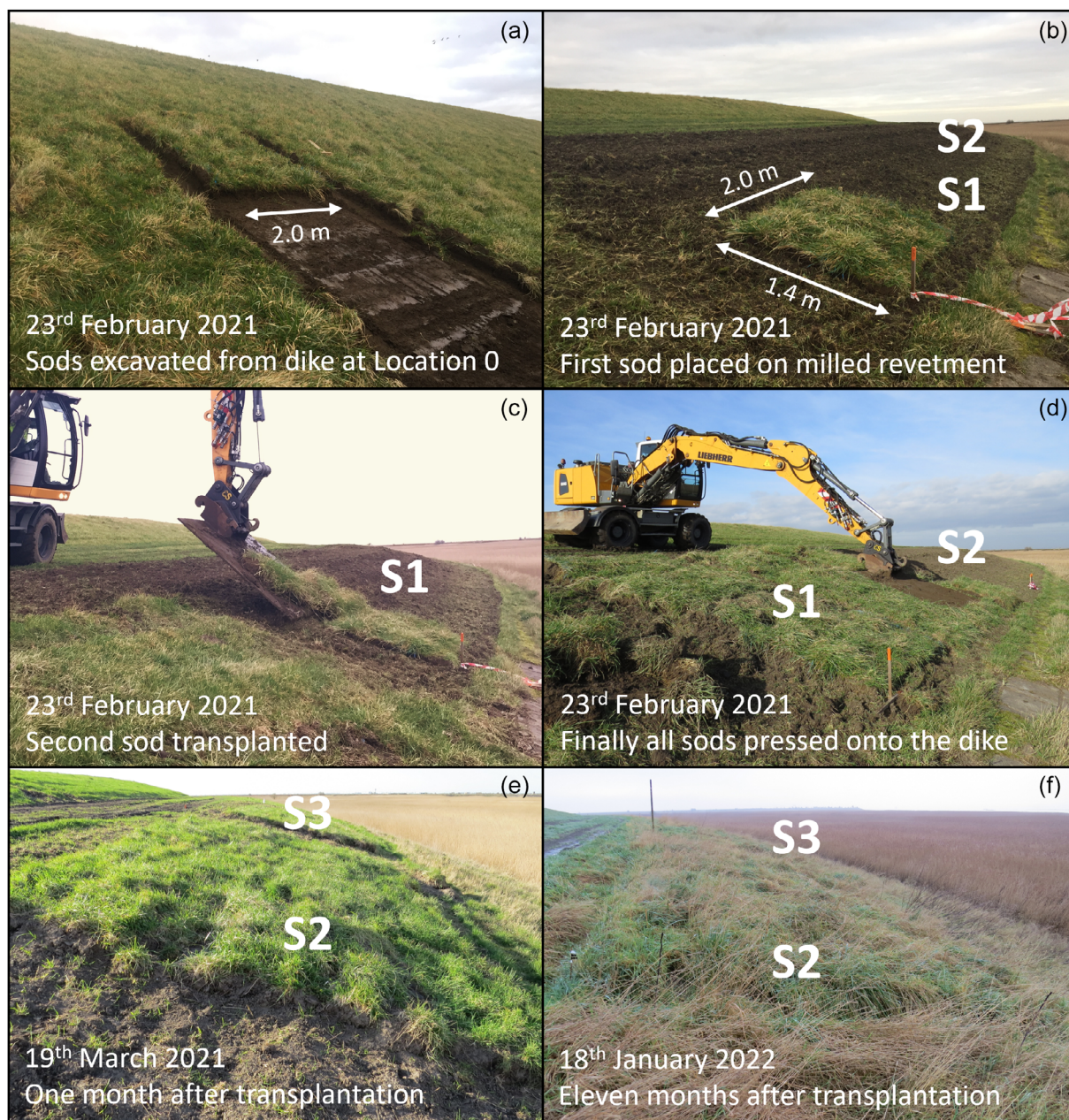
FIGURE 3 Grass sod transplantation technique. Grass sods excavated at Location 0 (a) and transplanted to experimental plots at the waterside dike slope (plot S1 in b, c, d and S2 in e, f). SodS were placed on the milled dike revetment (b, c) and pressed (d) to enhance firm connection with the dike. (e, f) Impression of sods plots after transplantation. Locations in Figure 1.
