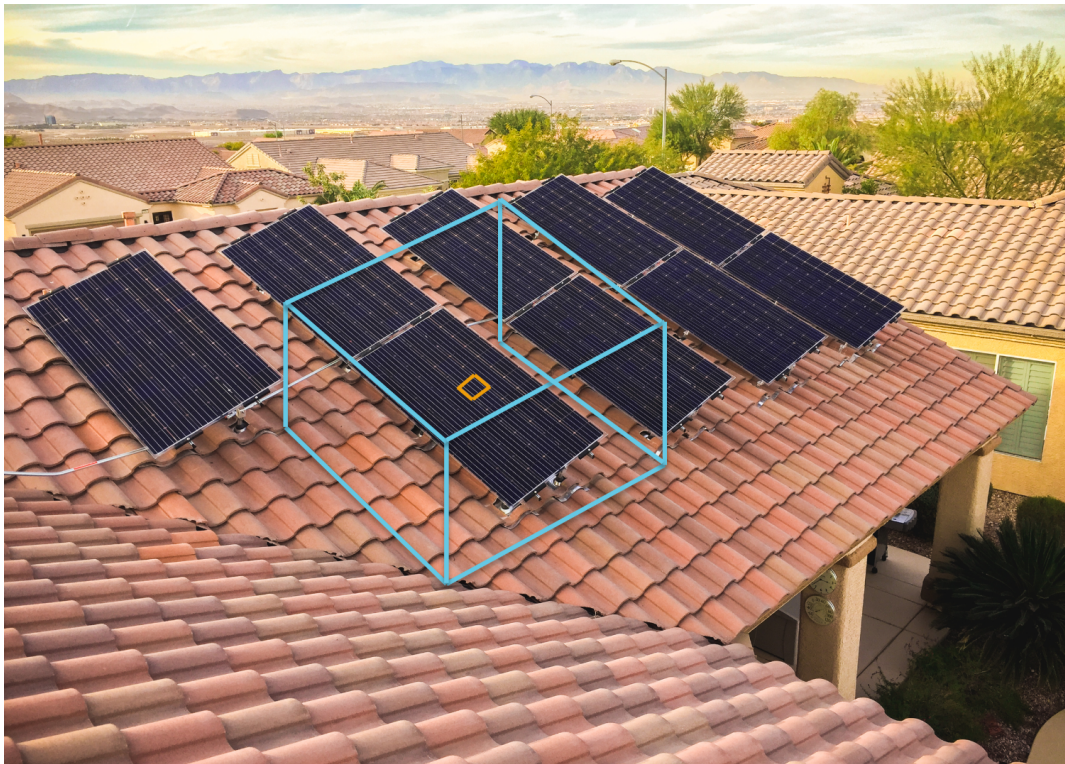
FIGURE 2.2: Example of a bifacial PV installation on a roof, where the space is separated in three units: Cell (orange), System Setup (blue) and Location.
