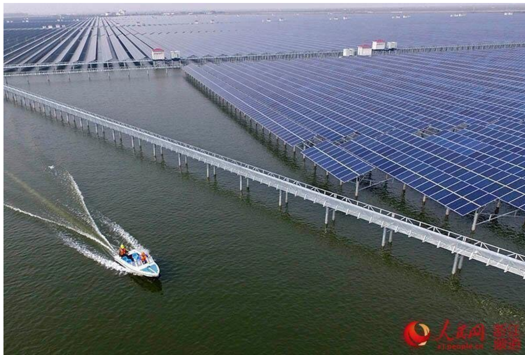
FIGURE 1.3: Example of a recently blossoming architecture PV module, bifacial PV; fulfilling a new application, floating PV; in a non-European location, China [3]
