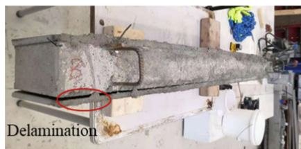
Fig. 6. Interface delamination for cast in-situ strengthened beam.
