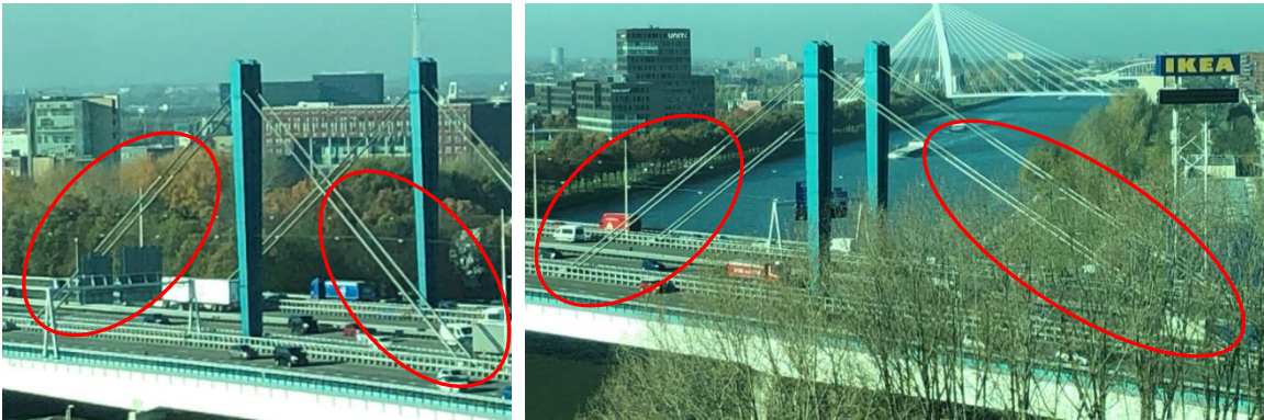
Figure 62 – Fire protection cover for the stay cables
