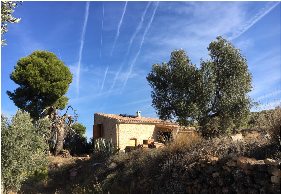
FIGURE 10 The barn after renovation
