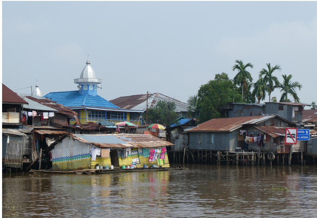
FIGURE 7 Building typology of riverine houses | Stilt houses and a floating house (left) at the junction between the Martapura and the Kuin rivers.
