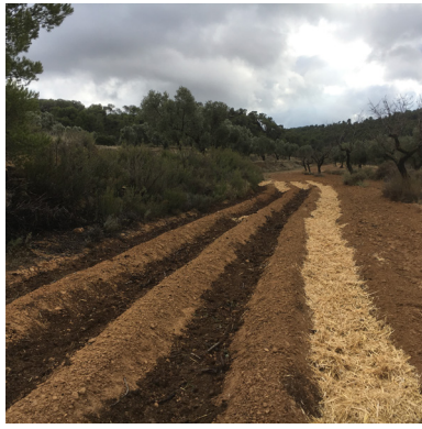
FIGURE 15 Preparing planting beds
