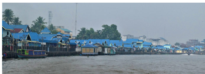
FIGURE 14 Kampong improvement project | One of the riverside kampongs - Kampung Biru - that underwent physical improvement or 'beautification.'
