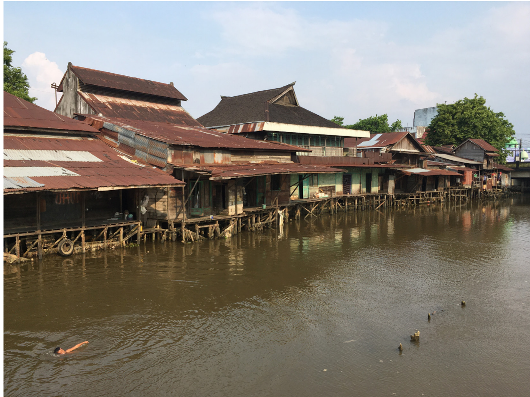
FIGURE 9 Riverfront of the old rice market | Riverfront of the old rice market, alongside the Kelayan river, displaying vernacular architecture features.
