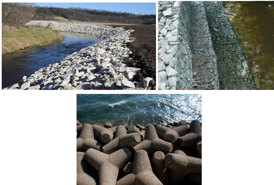
Figure 3.26, Figure 3.27 and Figure 3.28: Examples of rock and block armoring
