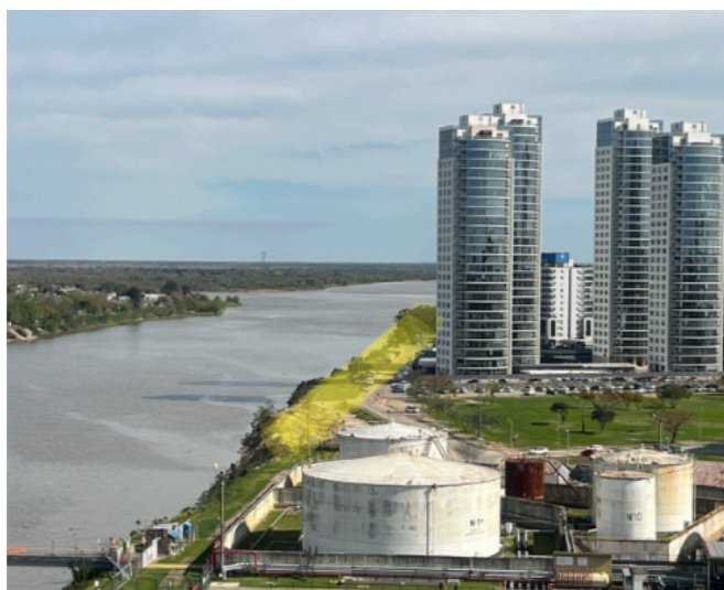
Figure 2.11: Project slope highlighted in yellow, located between residential towers and the Raízen oil storage terminal on Dyke 2
