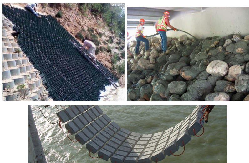
Figure 3.29, Figure 3.30, Figure 3.31 : Examples of armored slope blanket
