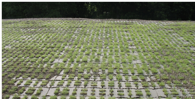
Figure 6.2: Articulated concrete block mattress (ACB)
