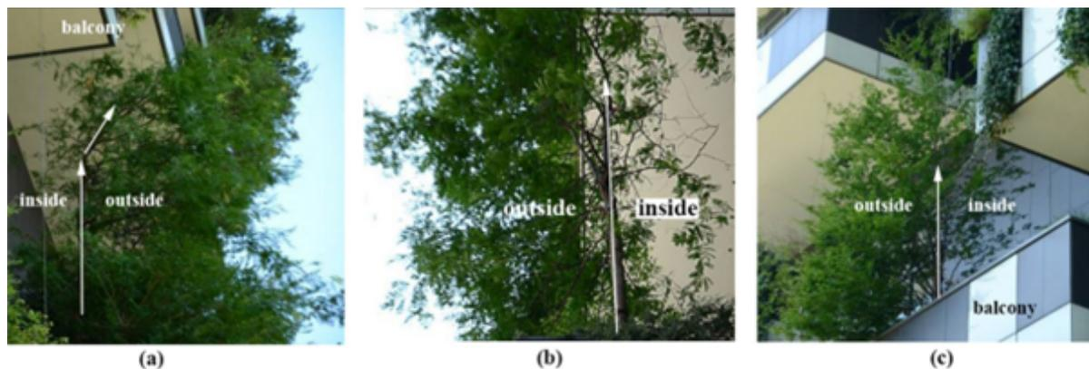
**Figure 6.3:** Growth of trees in Bosco Verticale, a) distorted stem and branches, b) and c) trees with different foliage density (inside near building surfaces and outside to the open air) [20]
