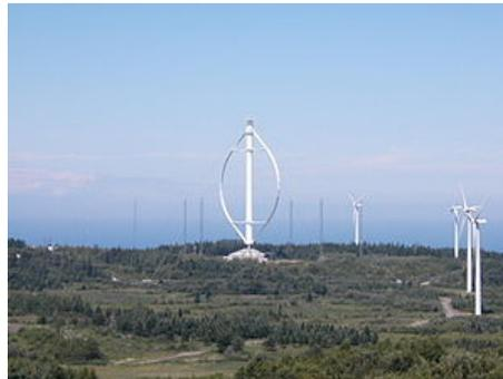
**Figure 1.2:** Eole, the 3.8MW Darrieus VAWT in Le Nordais
