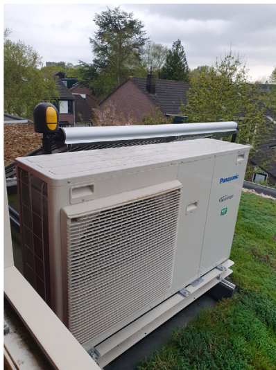
Fig. 2. View from the roof of the retrofitted house. From left to right: solar boiler, heat pump and sedum roof cover (picture by first author).
