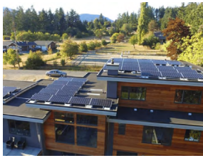
PV panels on the roof; public domain
