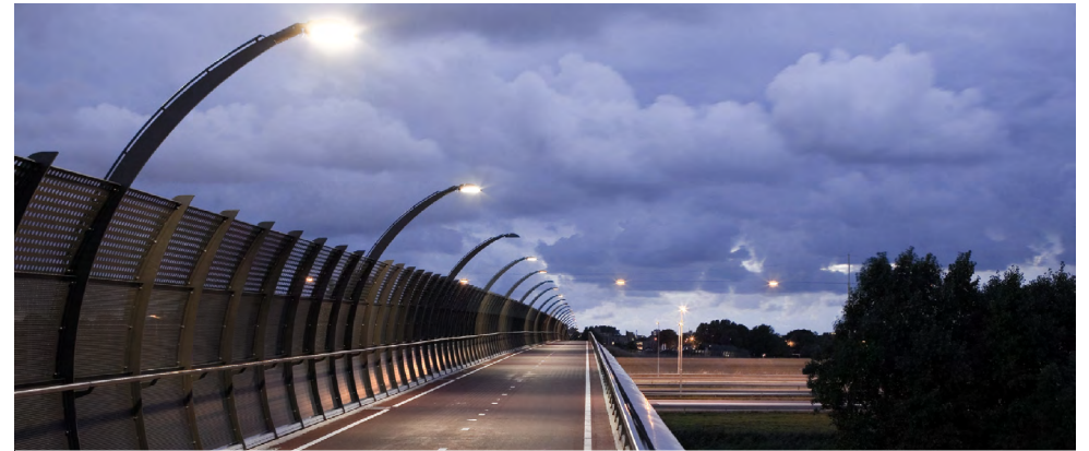
Image 79. Present condition of bicycle lane
