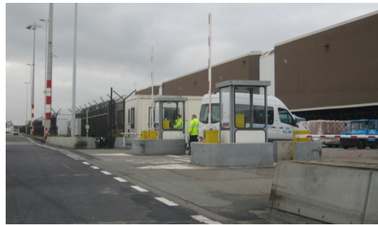
Figure 7.7; Photo of the KLM Cargo security post on the right side of the RH-road (main axis) (07-11-2012, 14:11:01 PM)
