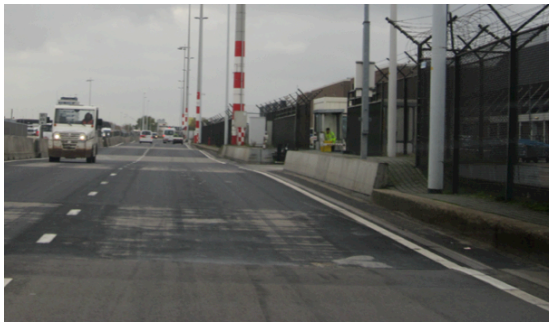
Figure 7.6; Photo of the RH-road (main axis) with possible space on the right side (19-09-2012, 14:10:23 PM)
