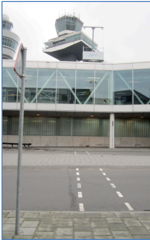
Figure 7.17; Pedestrian crossing, using channeling stripes, at the 'ACC building' (07-11-2012, 12:52:32 PM)
