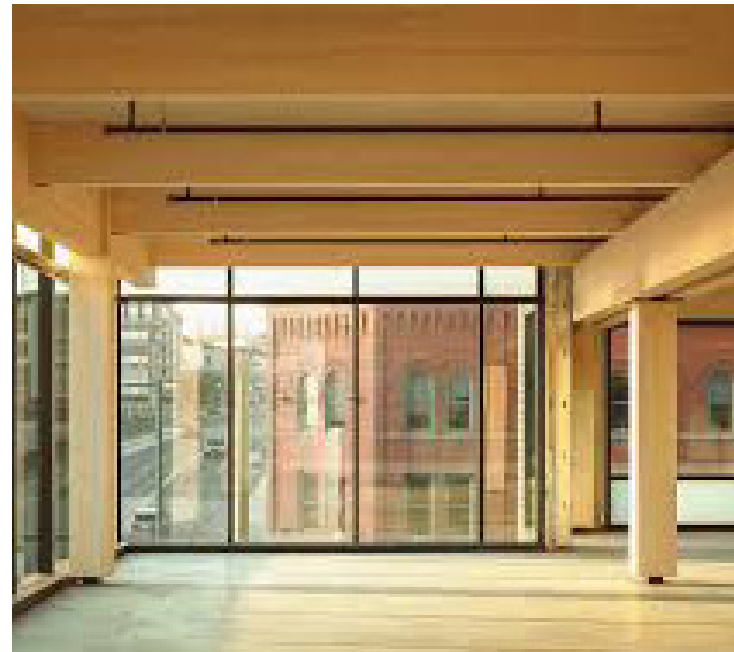
CLT & Glulam construction with black steel connections
