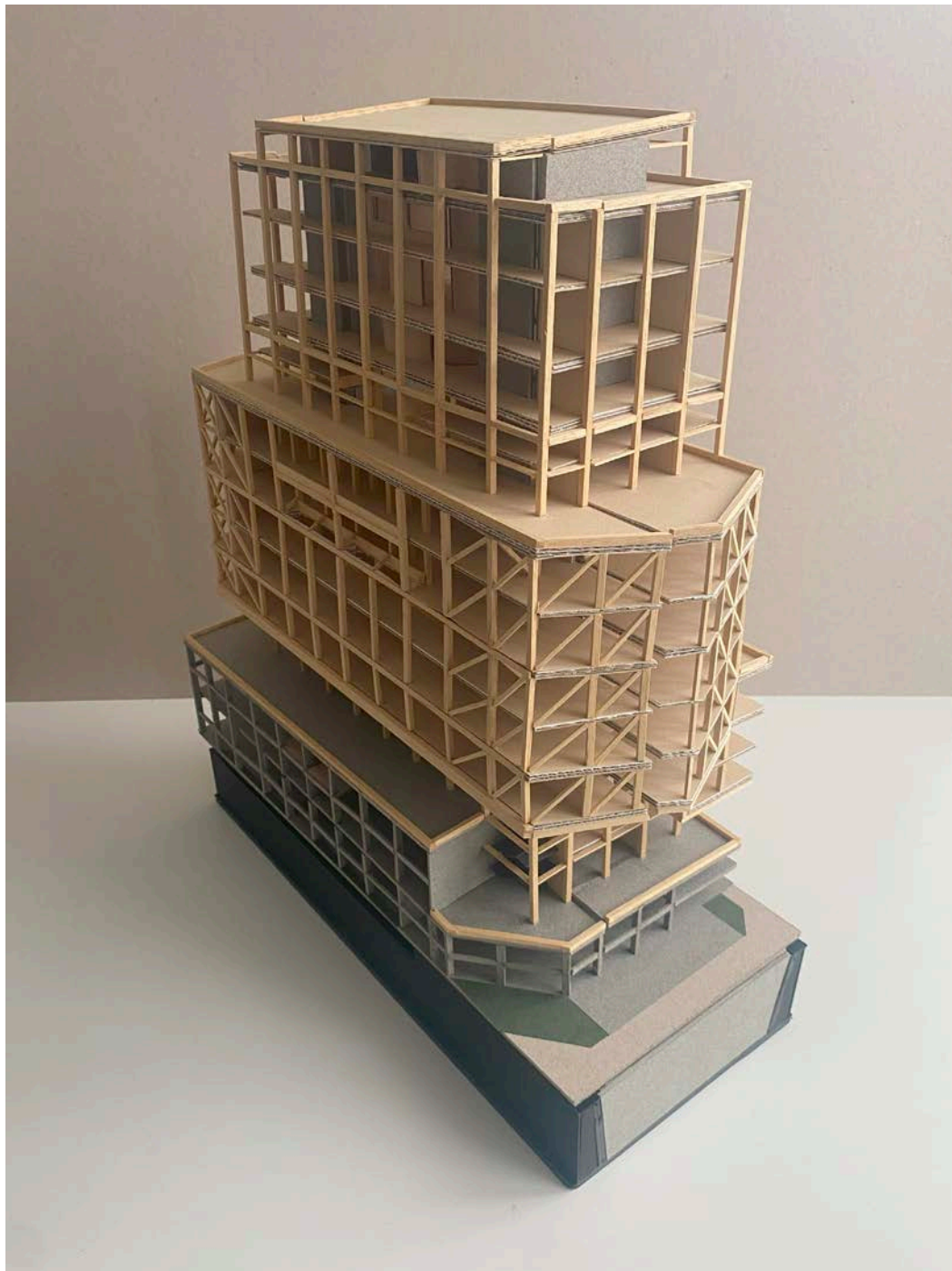
Timber structure, concrete foundation, and concrete cores
