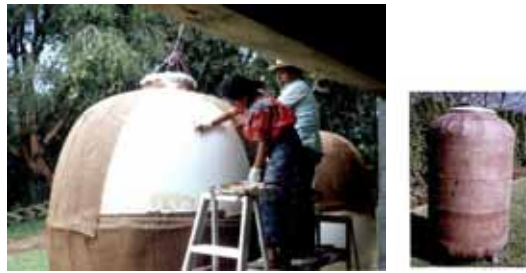
Figure 6.1: Construction of water tanks with biocomposite in Guatemala [van Rijswijk et al., 2003]
