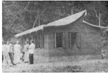
Figure 10.3: Ferrocement roofs for houses by Arobindo Ashram in India [Paul and Pama, 1978]
