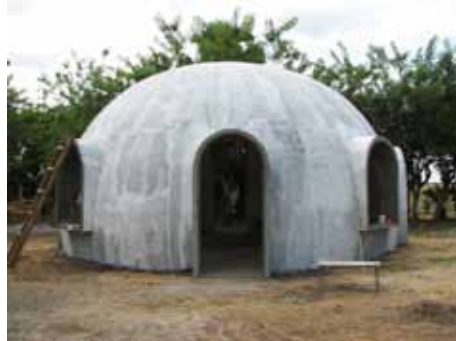
Figure 10.27: While lower meter of the inflatable formwork was vertical, the resulting shell bulges outward [Viguurs].
