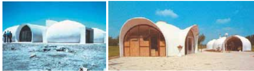
Figure 4.16: Isler, prototype for housing project in Iran and 'balloon shells' in Ponthierry, used as work studios. [Hennik, 2005]
