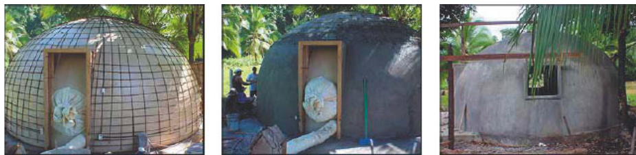
Figure 4.23: Construction of an 'Ecoshell' [Hennik, 2005]
