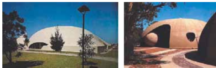
Figure 4.17: left: Binishell on rectangular base (Randwick Girls High School, New South Wales, Australia). right: Binishell on circular base (The North Narrabeen Primary School, New South Wales, Australia). [Hennik, 2005]
