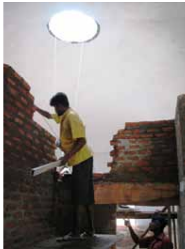
Figure 11.46: Building brick walls in the first dome in Inspector Eatham, Sri Lanka. [Viguurs]
