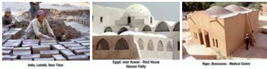
Figure 4.4: Adobe, production and construction [Auroville, 2006]
