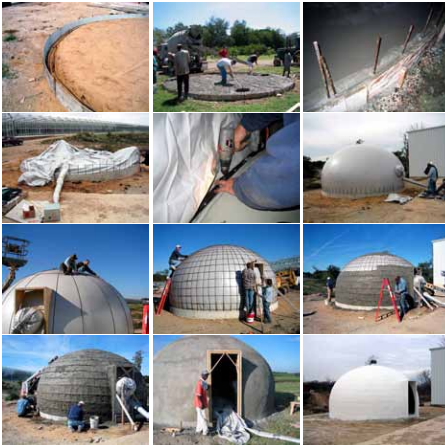
Figure 2.2: Building process SolidHouse and MDI [MDI, 2005]
