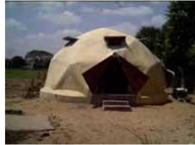
Figure 6.4: Ferrocement Geodesic Dome in Sri Lanka [geocities, 2006]
