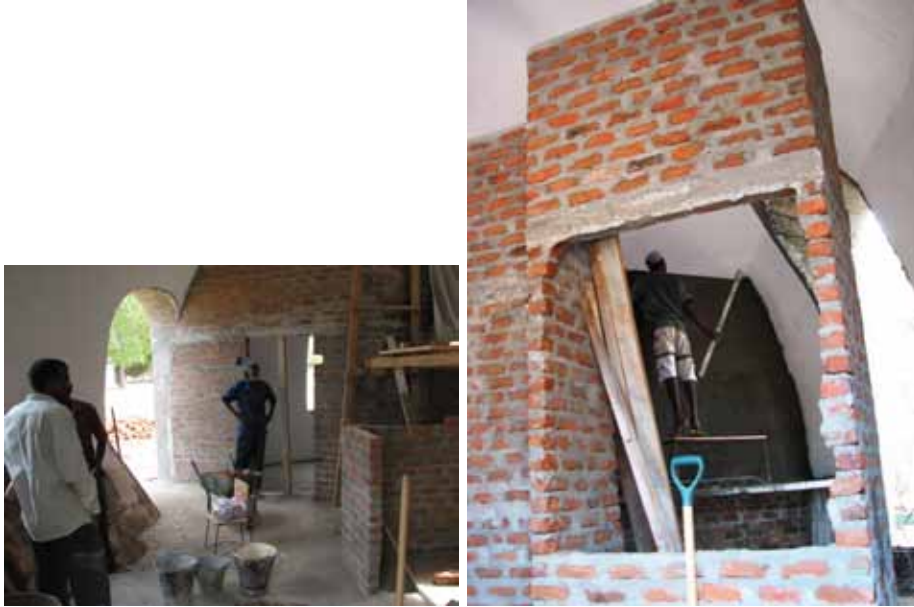
Figure 11.33: Inner walls built with 'home-made' CSEB's (see section 6.4) in the first dome in Inspector Eatham [Viguurs].
