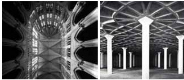
Figure 4.11: Ribs in building engineering: Amiens cathedral [Portoghesi, 2000] and Nervi's Getti Wool Factory [Otto and Others, 1982]
