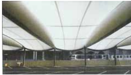
Figure 11.20: The permanent roof of a parking garage in Montreux (Switzerland) is supported by inflatable girders [Lombardi, 2006].
