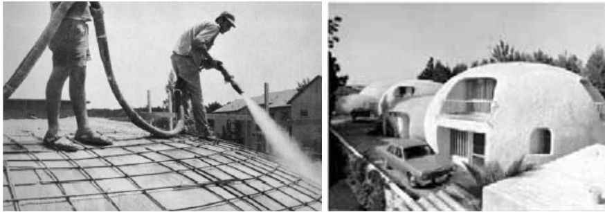
Figure 4.14: Heifetz, left: Applying shotcrete on inflated formwork, right: Villas in Ramat Hasharon, Israel [Hennik, 2005]
