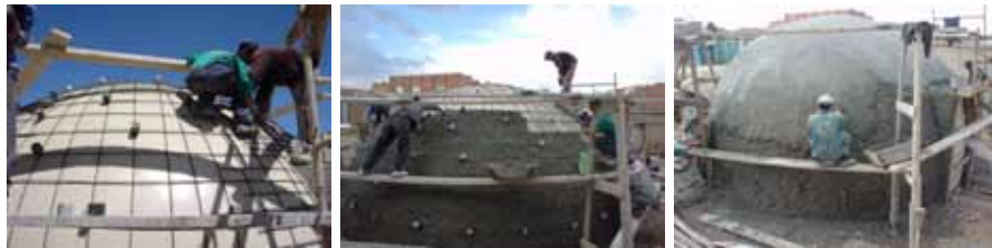
Figure 2.3: Building SolidHouses in La Paz, Bolivia [SHF, 2005]
