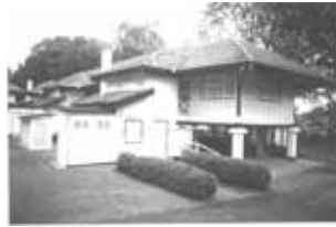
Figure 7.3: In these colonial bungalows in Singapore the most important function of the roof is to provide shade and protect the walls, allowing skin cooling through the use of lightweight materials. The large overhangs allow the windows to be left open in case of rain, allowing ventilations at all times except in storms. [Hyde, 2000]
