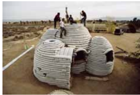
Figure 4.30: Dome built with superadobe system of Khalili [Calearth, 2006]
