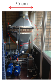
Figure 3.6: The installation of the tube-fin air cooler surrounded by a red circle. The two horizontal headers used to distribute the flow of hydrate slurry into 15 parallel circuits is clearly visible. Each vertical row of tubes is a different circuit.
