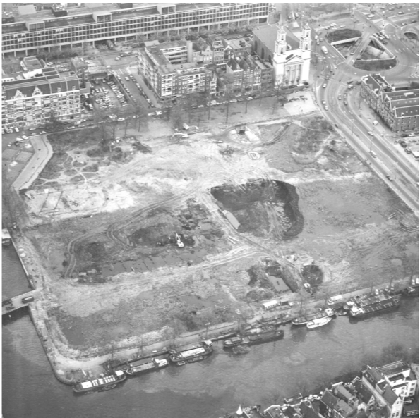
Construction 1980 New plans for a metro line removed Vlooienburg completely
