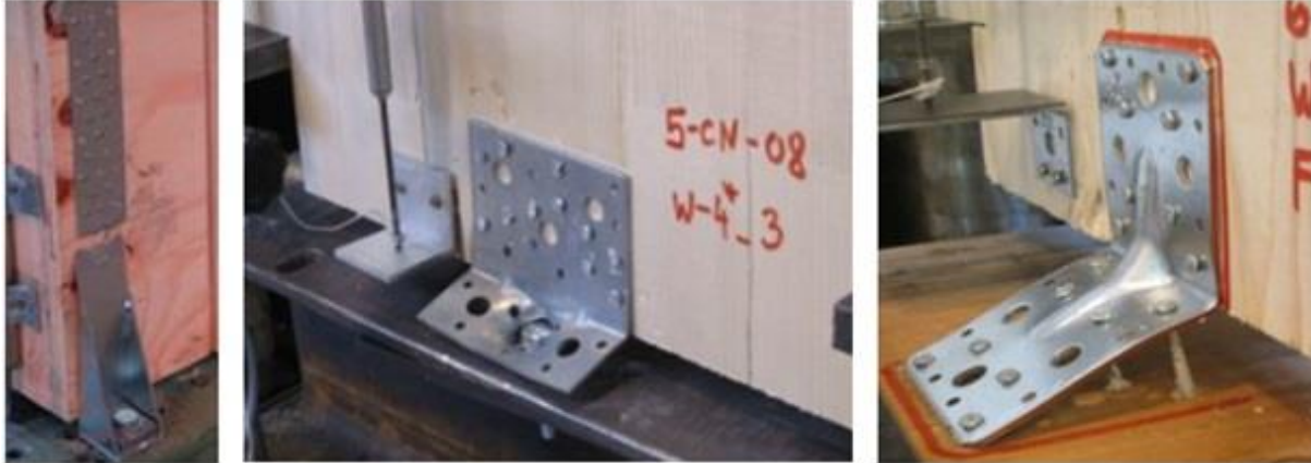
Fig. 3.22 Brittle failure modes of CLT connections: failure of steel hold-down, pull through of the bolt in the steel part of the angle bracket and yielding of the steel part of angle bracket with nails withdrawal. (Gavric, Fragiaco, & Ceccotti, 2013)
