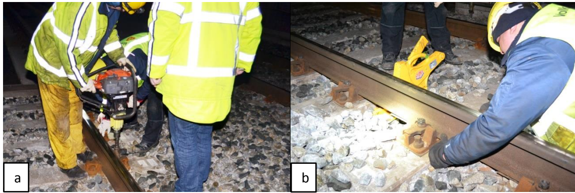
Figure 12. Adjustment of the fasteners.
