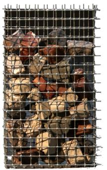
Reclaimed bricks from the crumbling bunkers are gradually filled into the gabion.
