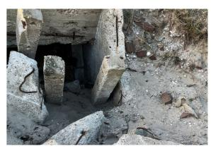
Figure. 56-58 Bunker ruins in the dune. The Atlantic Wall bunker in the dunes is gradually becoming ruined, invaded by vegetation and structurally damaged. (photo by Flak Gruko, 2016)
