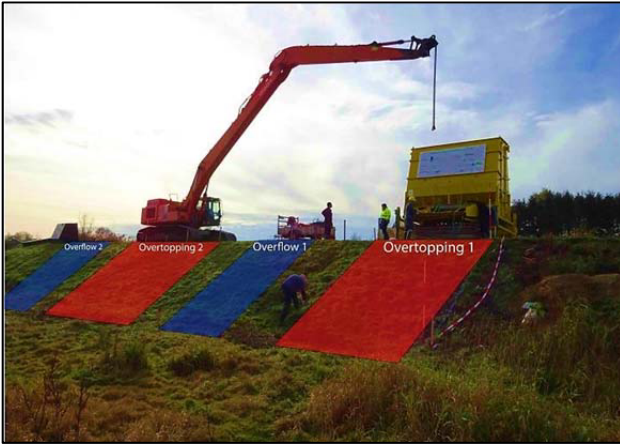
Figure 1. Overview test locations on embankment.
