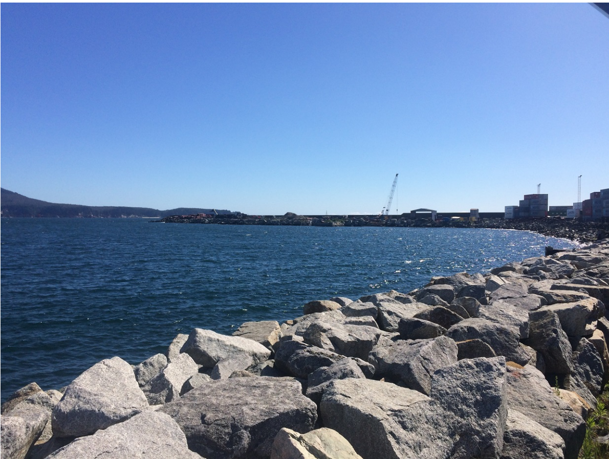
Figure 8.1: Between the breakwater and the container storage area, a small bay is present. This sheltered area can be an attractive location to start an expansion. It is protected by the breakwater and close to the quay.
