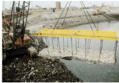
Figure 3.12: Crane placement
