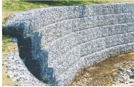
Figure 2.9: Soil retaining wall
