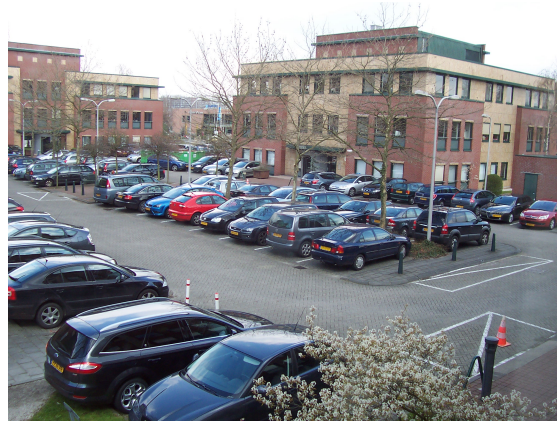
Figure 5.1: The Logica building, located in Rotterdam
