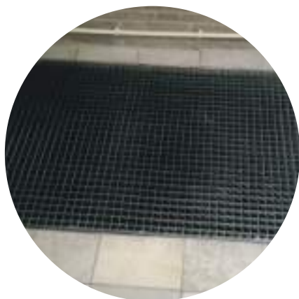
Figure 226 Grille for the extraction of cold air.
