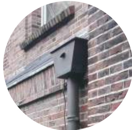
Figure 240 Downspout.
