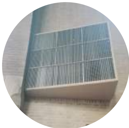
Figure 225 Air vent for warm air.
