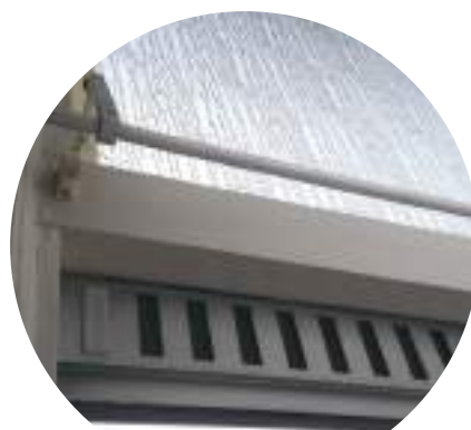
Ventilation grille above the window.
