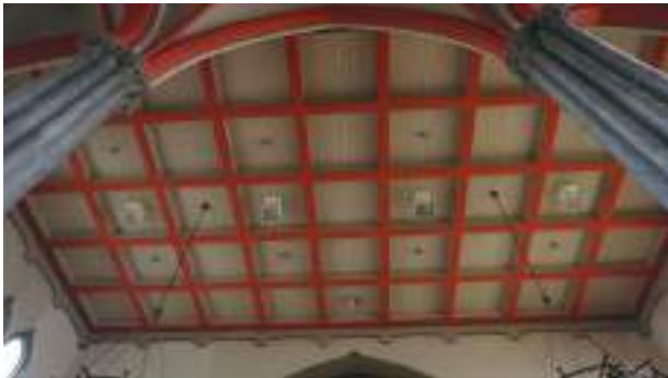
Figure 2 The ceiling of the new part is made of softboard which has good acoustic qualities.
