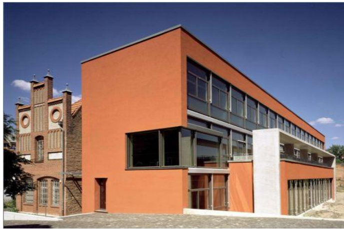
Figure 1. Test Case Building, Kassel Germany.
