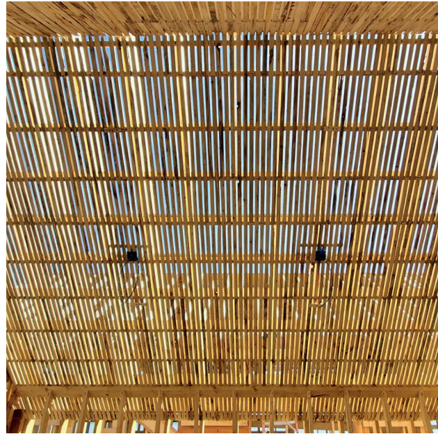
2) Reed matting is secured to the timber (inner side) for capturing the spray applied mixture
