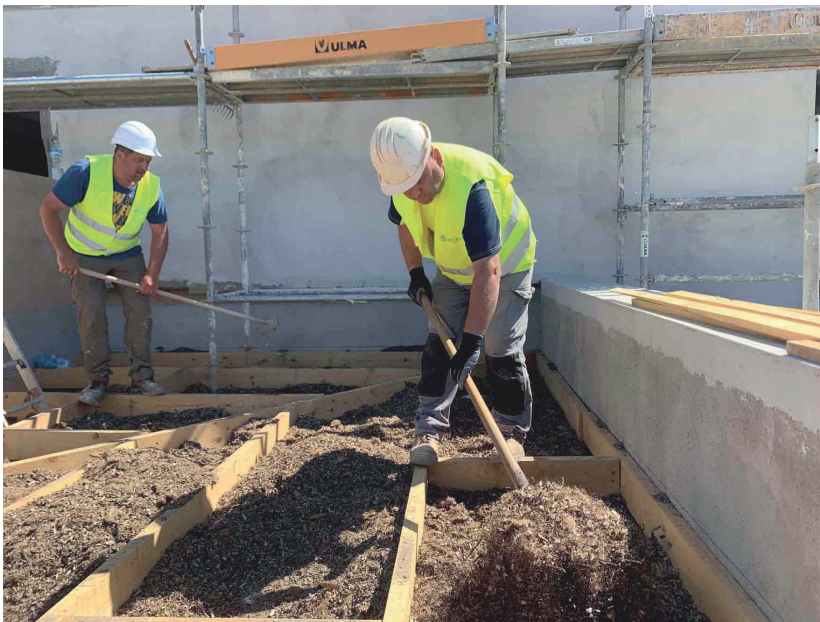
15) Workers distribute and level the locally-sourced 'Posidonia oceanica' seaweed insulation within the roof assembly framework.
