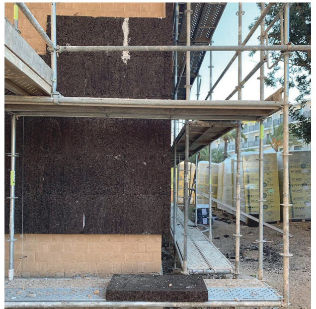
16) The cork-based insulation panels are screwed to load-bearing CEB walls, before a lime plaster finish is applied.
