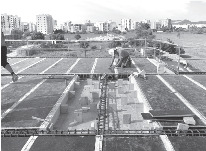
11) Wooden blocks and boards are also laid out for the formwork, for the concrete to be poured over to form the soffit.
