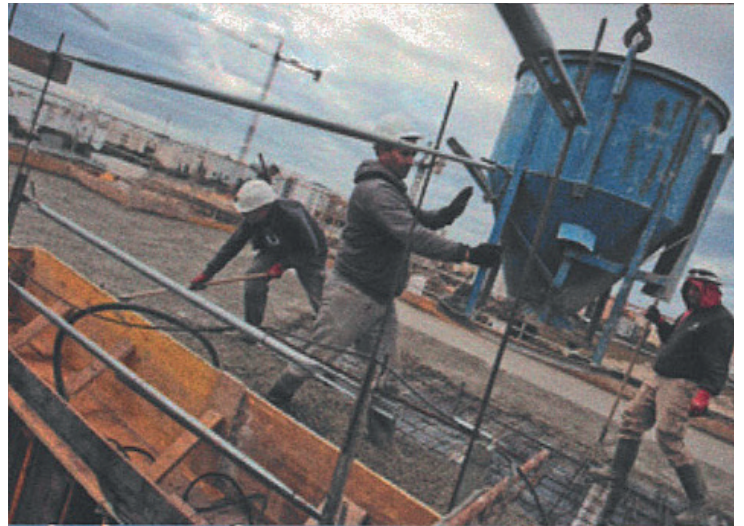
12) Concrete is poured into formwork using a concrete bucket attached to a crane. The steel reinforcement bars can be seen getting filled.
