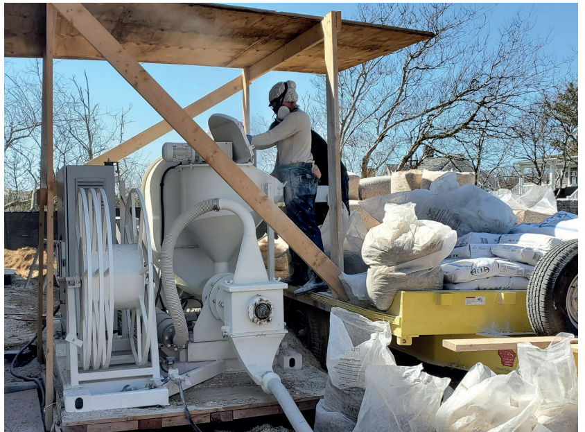
4) In the Valkyrie, a French Hempcrete Spray Machine, hemp shivs are mixed with lime and water
