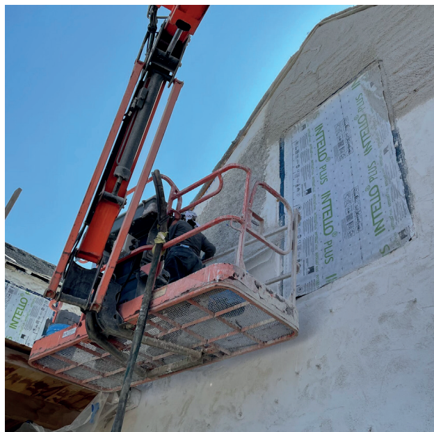
6) After drying, plaster is spray-applied to walls, using the JLG boom lift
