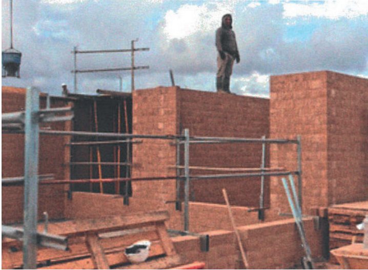
9) Workers finish constructing the vertical walls to their full height, preparing for the integration of structural floors or roofs.
