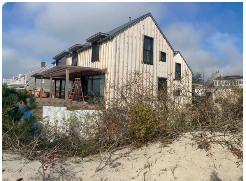
7) Square timber spacers are added in intervals to get the alignment right and then wooden vertical and horizontal battens are screwed on, ready for shingles to be nailed on.
