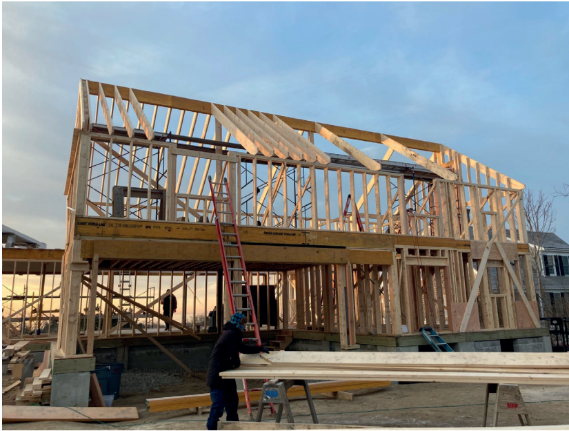
1) Timber wood structural frame goes up
