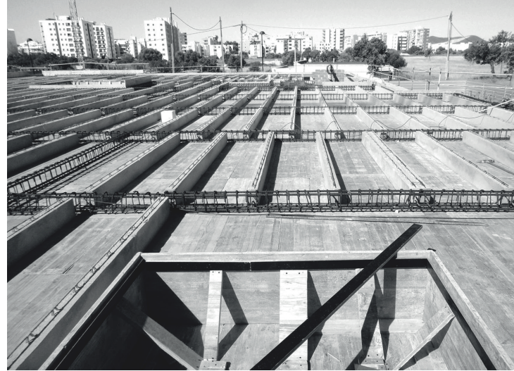
10) Assembly of precast floor system where precast concrete beams and hollow-core blocks are laid out on a structural framework for the floor slab.
