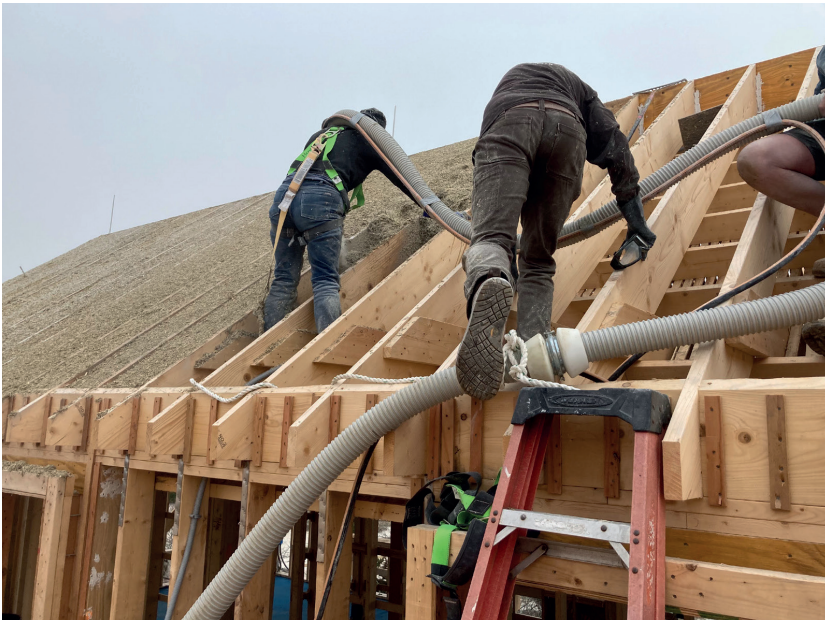
5) Hemplime mix is sprayed onto the roof
