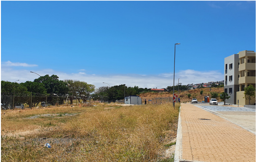
Setback to (new) Hanover Street and Phase 3 redevelopment
