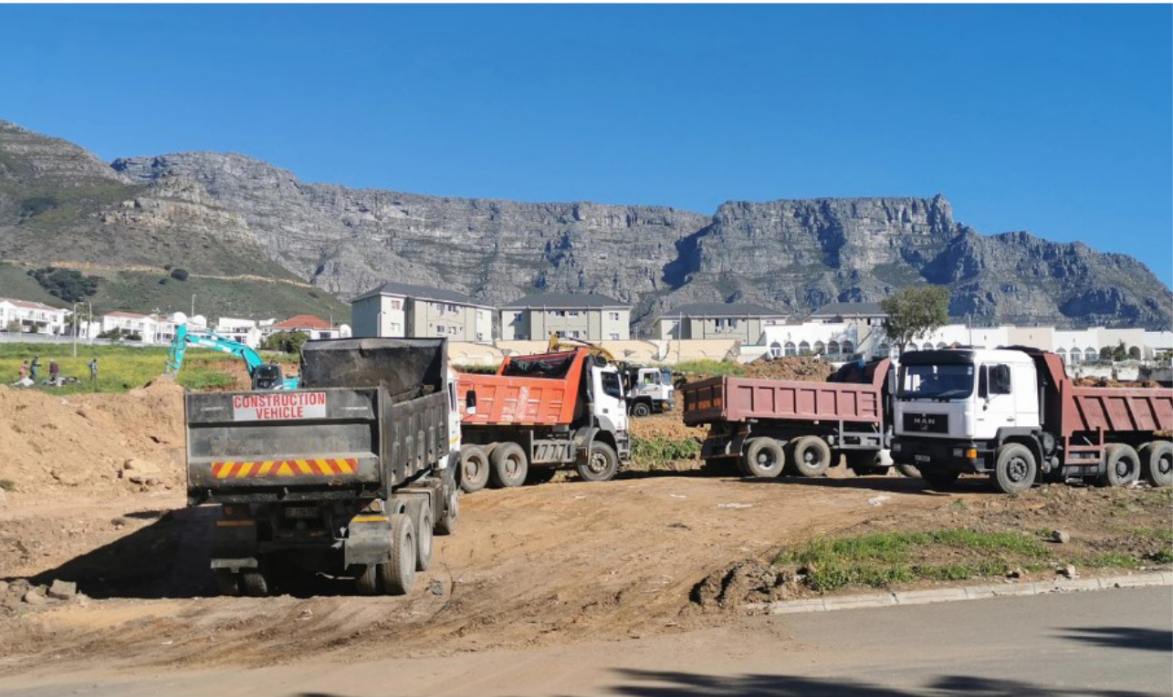
Trucks and bulldozer in District Six. (Photo: Sune Payne)
