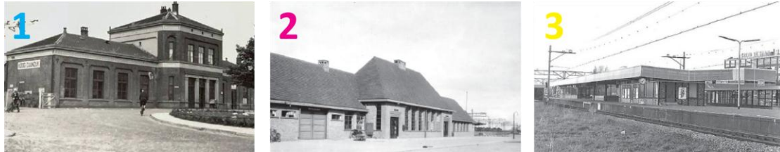
Figure 17: The 3 station buildings of station Koog-Zaandijk
