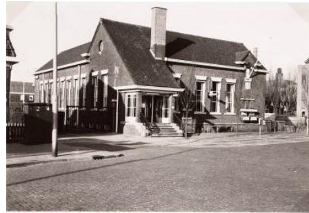
Figure 27: Former Post office
