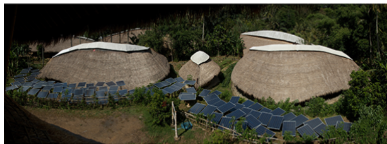
Figure 1.3: Implemented Off-grid Project (copyright of UNDP Indonesia)
