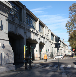
5 View of a tunnel running below the tracks, featuring three entrances and 8-meter-high walls.
