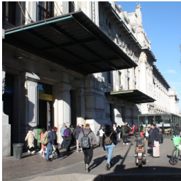
4 Side indoor entrance with an external weatherproof roof extension, and a new restaurant structure visible in the background.
