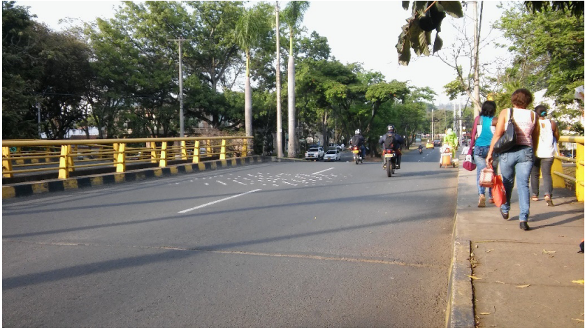
A. Bridge traffic flow view
