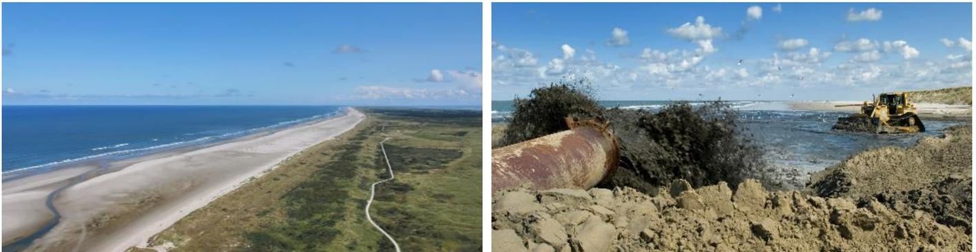
Figure 1 Sandy beach with vegetated dunes (left panel) and sand nourishments being carried out on the beach through pipes (right panel) in the context of Dynamic Preservation, on the north side of the Wadden Sea Island of Ameland, The Netherlands. From: "Kustonderhoud Waddeneilanden", source: Rijkswaterstaat, n.d. Public domain (CC0)
