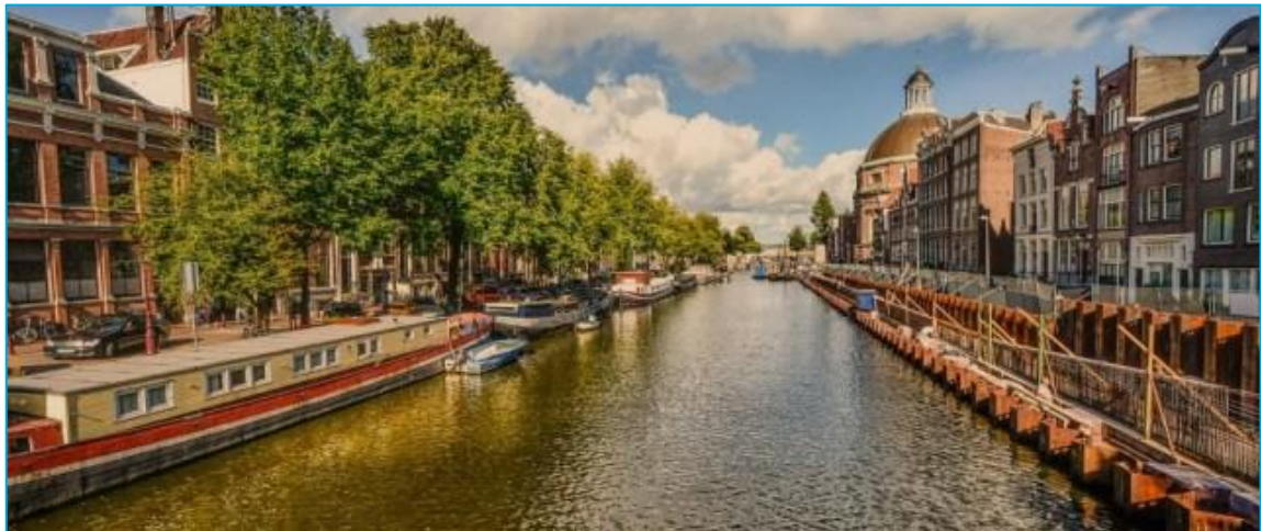
Figure 4 - Temporary sheet pile quay wall (SkyGeo, 2024)
