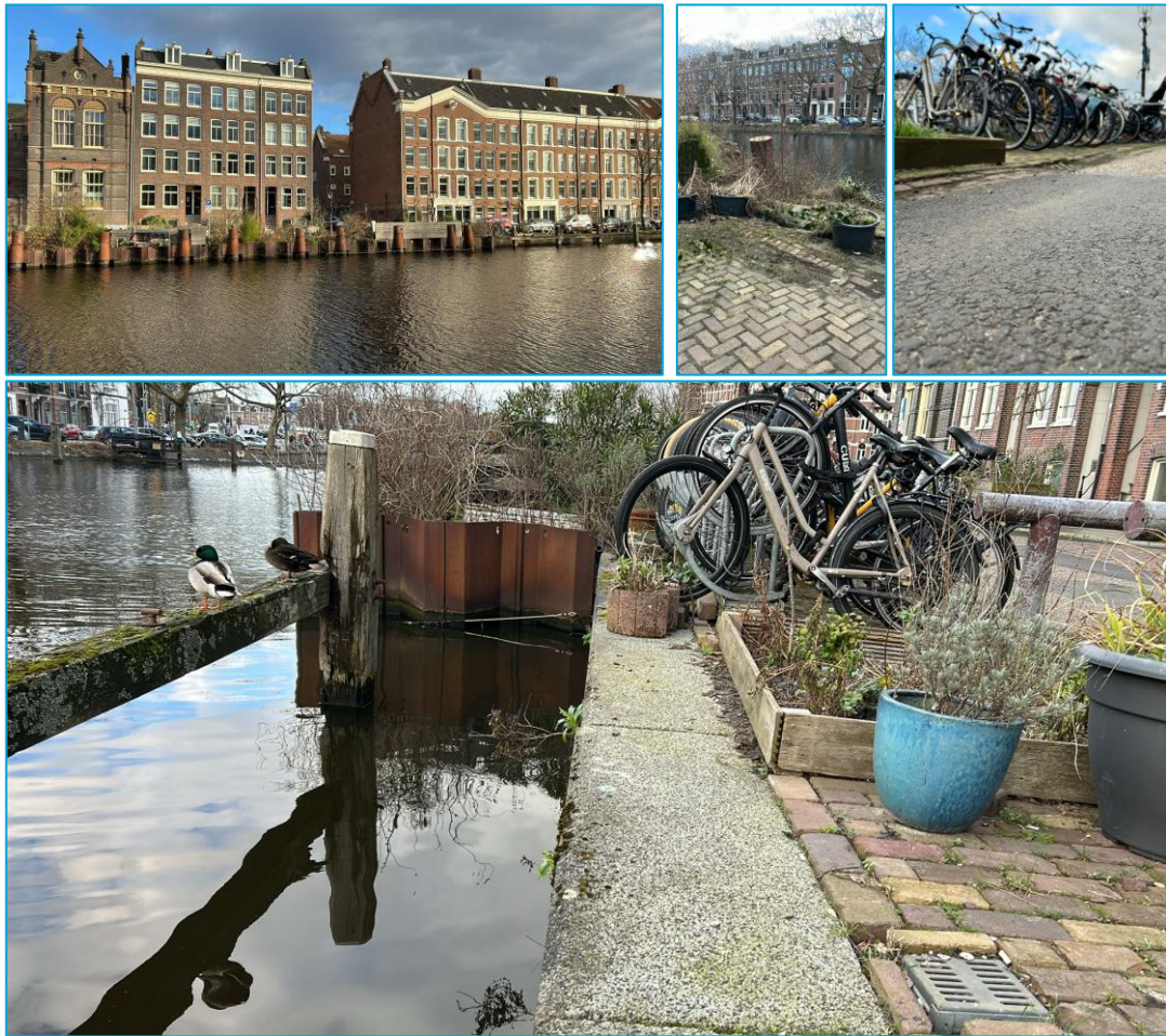
Figure 79 - Photos of the steel support structure of the Marnixkade and local settlements (van Vliet, 2025)
