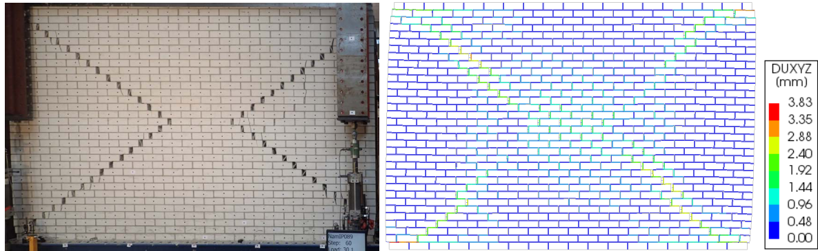
Figure 6.4: Observed crack pattern in experiment of test COMP_4 and the absolute value of relative displacement of the interface in deformed mesh for COMP_4 (scaling factor=10)
