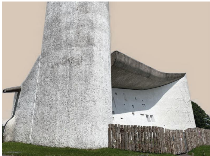
Figure 19: South façade of the chapel
