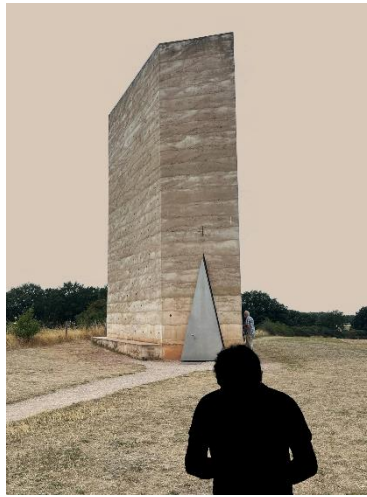
Figure 3: Investigating the chapel
