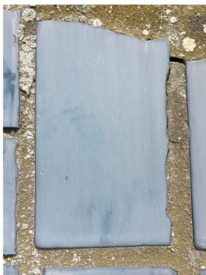
Figure 3. Detail of the lantern's exterior showing one dalle de verre slab with a residual coating of the 1990s remedial polymer treatment and, surrounding it, the embedding epoxy mortar with a prominent gap at the upper right. Courtesy of Norman Tennent
