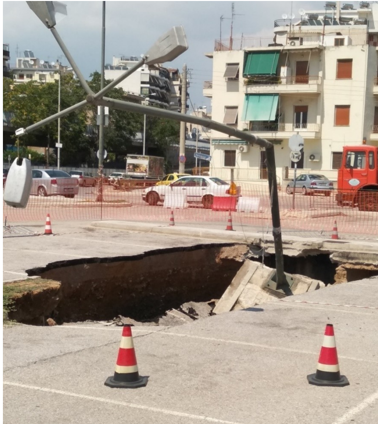
Figure 6-14 Land subsidence at parking slots over Ilissos, 2018 (photo by the writer)
