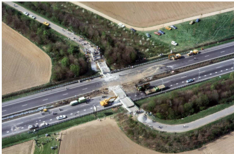
Figure 1. Aerial image of a collapsed viaduct 'KLEINE HEIDE', the Netherlands 22 APRIL 1987.
