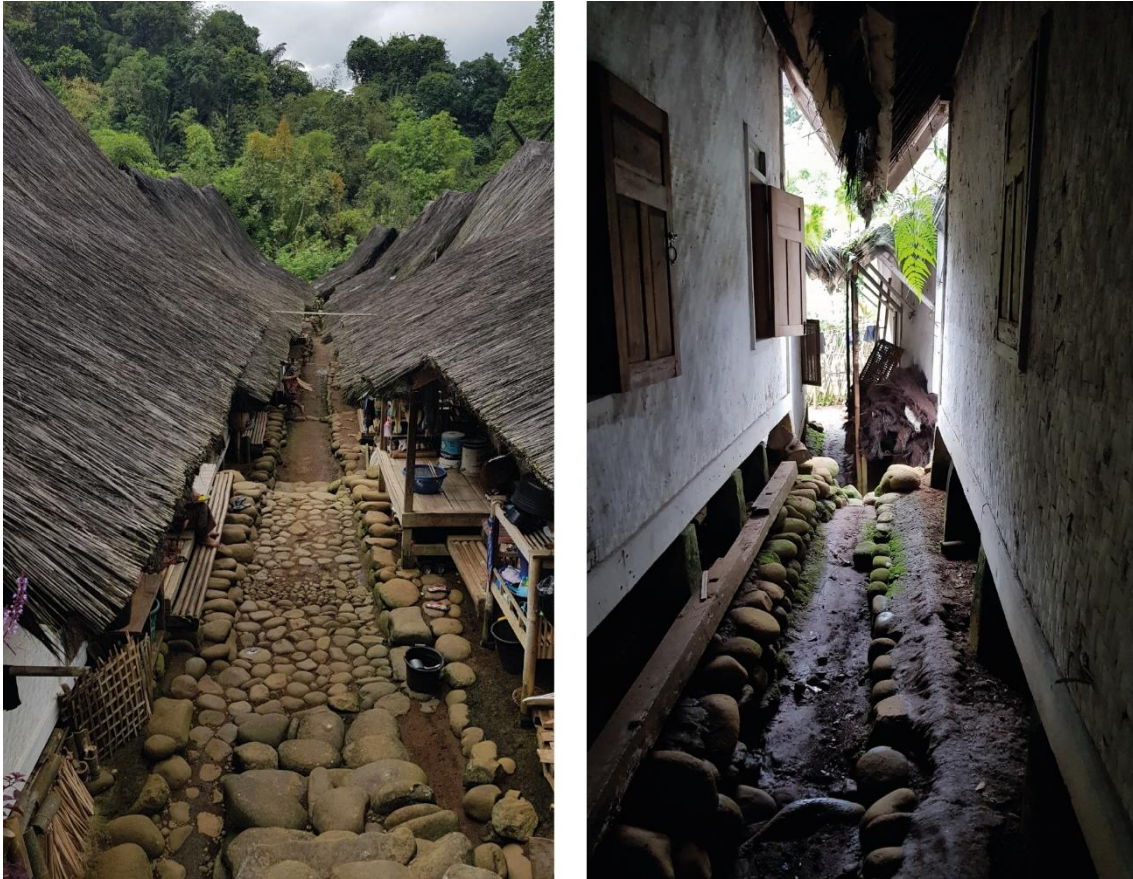
Figure 66. Narrow passages shaded by significant overhangs provide cooling in Kampung Naga. (Images by author.)
