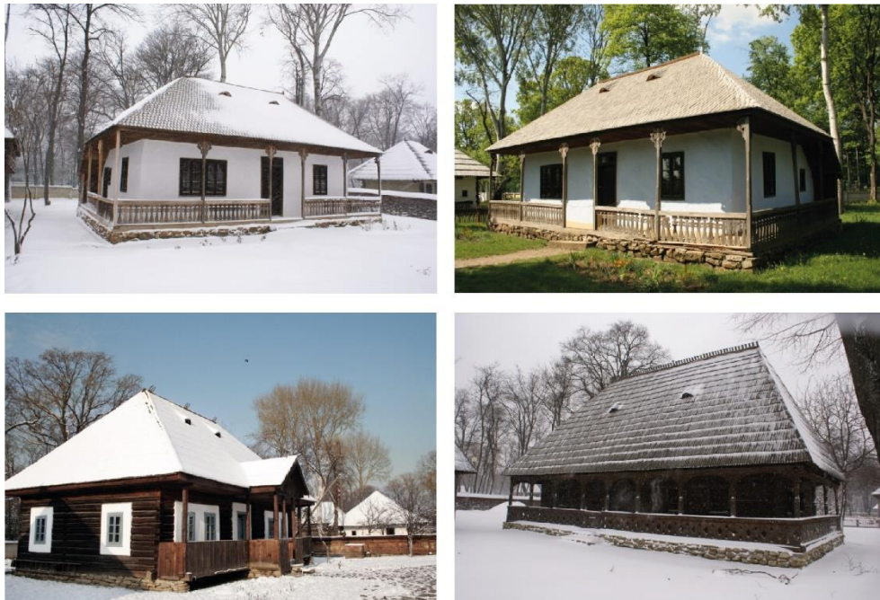
Figure 52. Traditional Romanian buildings with low stone foundation and verandas. (Retrieved from: http://muzeul-satului.ro/ )
