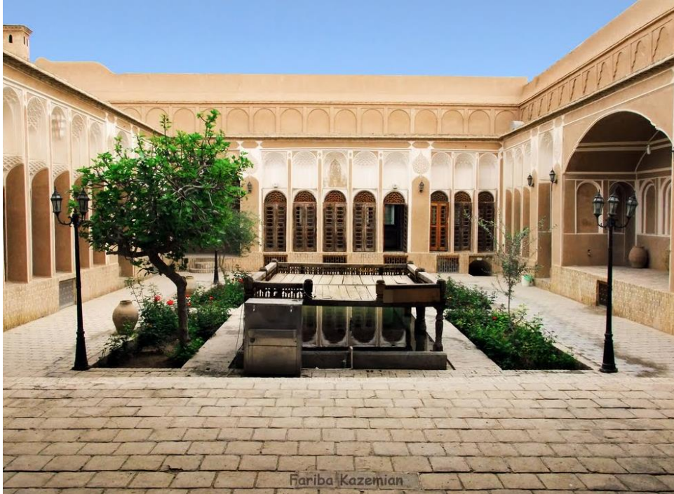
Figure 58. Courtyard in Yazd. In front higher west or east facade with openable shutters and windows. On the sides arcades providing shade and heat buffer. (Retrieved from: http://www.panoramio.com/user/4082241?with_photo_id=55969042 )
